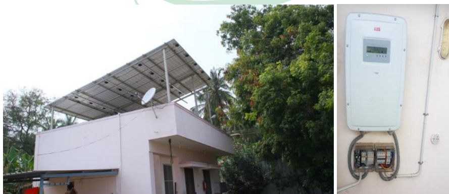
Installation of 5.5kWe solar photovoltaic and net metering system
