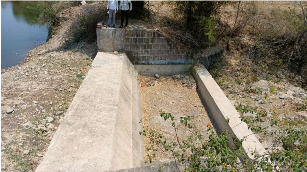
Constructed Check Dam. Babina block of Jhansi district
