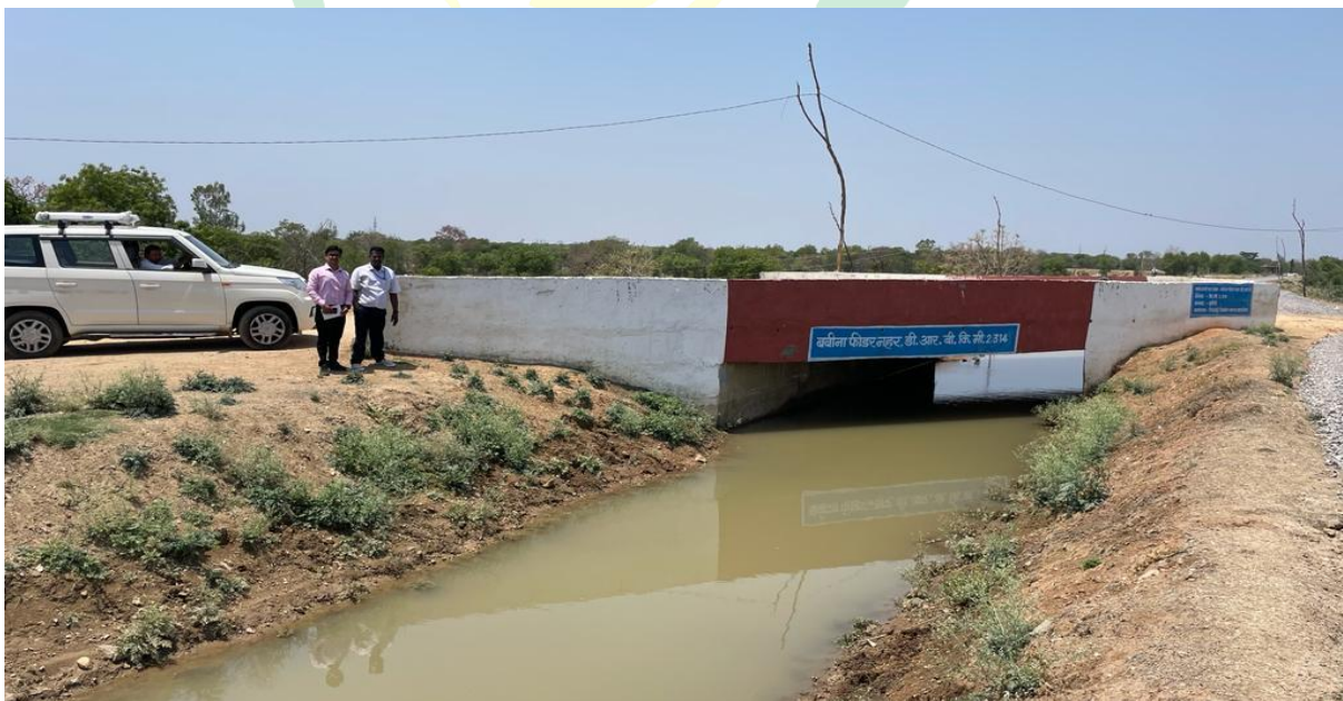
Main Channel from Betwa river
