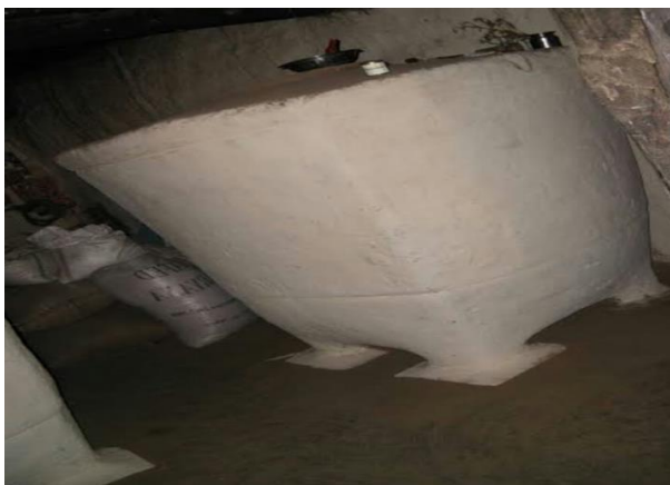
Fig. 1. Grains storage structure (Dholi)
