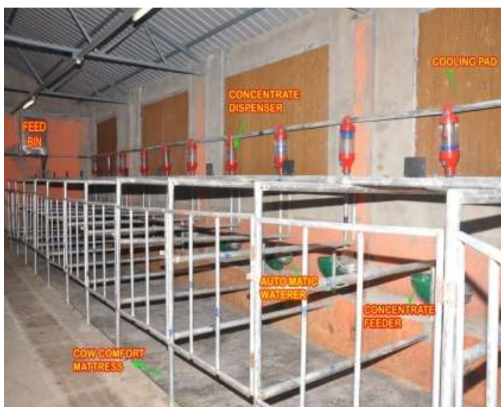
Illustration: I Model of Environmentally controlled Dairy housing system
